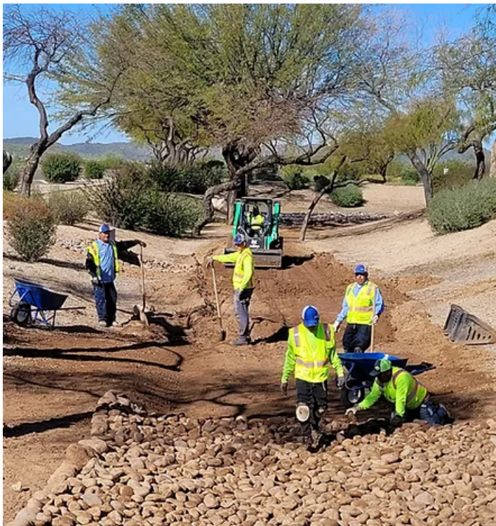
SDL working on erosion project
